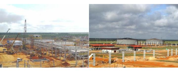
**Description:** Increase the capacity, either at the Plant and Heavy oil crude oil storage. Development of Detailed Engineering for Procurement and Construction of the new dehydration and desalination Trains of diluted wet bitumen streams, the diluted wet and dry bitumen storage and treated water arising from dehydration for the well injection.
